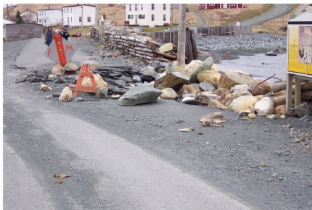
Photos from Coastal Erosion in Newfoundland Community Reports for Ferryland (left) showing overwash damage and and Humber Arm (right) showing a mixed gravel-sand flat.
